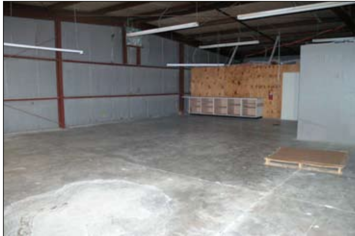
This is a portion of the warehouse at the 21st Street Building that will become part of Dayton-Superior production area.
